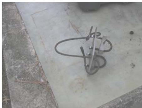
The mast we were installing was 20 feet long, weighing about 100 pounds. The haul rope was attached about 8 feet from the bottom of the mast. I had a muffler clamp there for some extra insurance to make sure the rope wouldn't slip.
