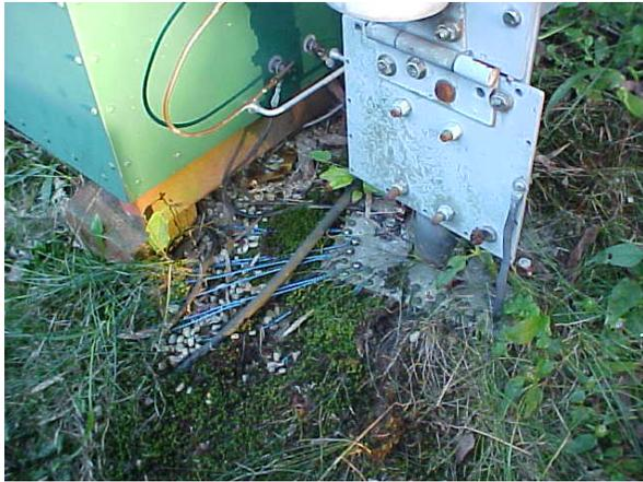
**Radial wires connected to aluminum base plate**
