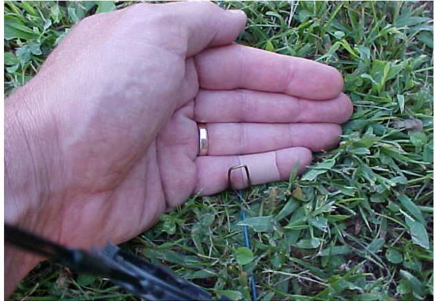
**A partially installed staple over a radial wire**
